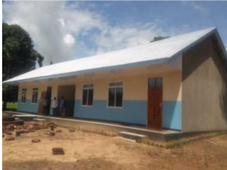
Figure 12: Magereza Primary School double classrooms built and office with funding from the Community, Government, and KVTC Social Fund.
